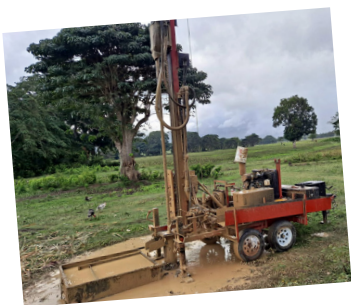
Drilling rig gets the job done!
